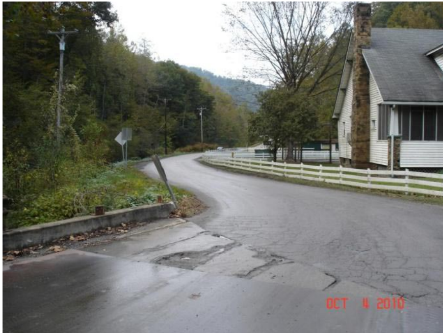
Picture 2: Northbound curve exiting bridge
