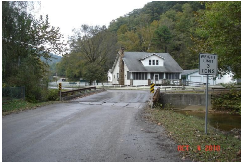
Picture 1: Existing deck condition
