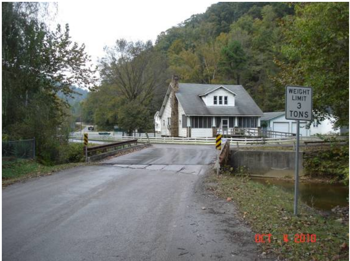
Photo of Bridge over Red Bird Creek
