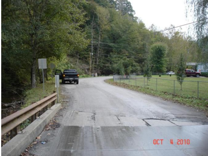
Picture 3: Southbound curve approaching bridge
